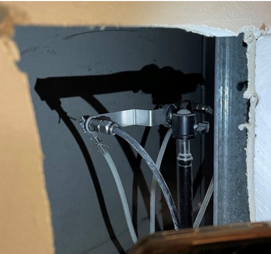
Fig. 5 - Sealing Station Spray Nozzles in Exterior Wall Cavity
